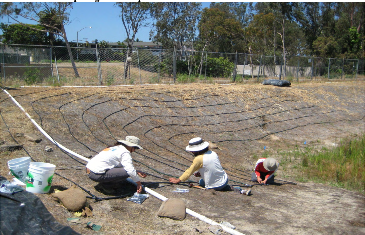
Photo 12. SMS drip irrigation setup
