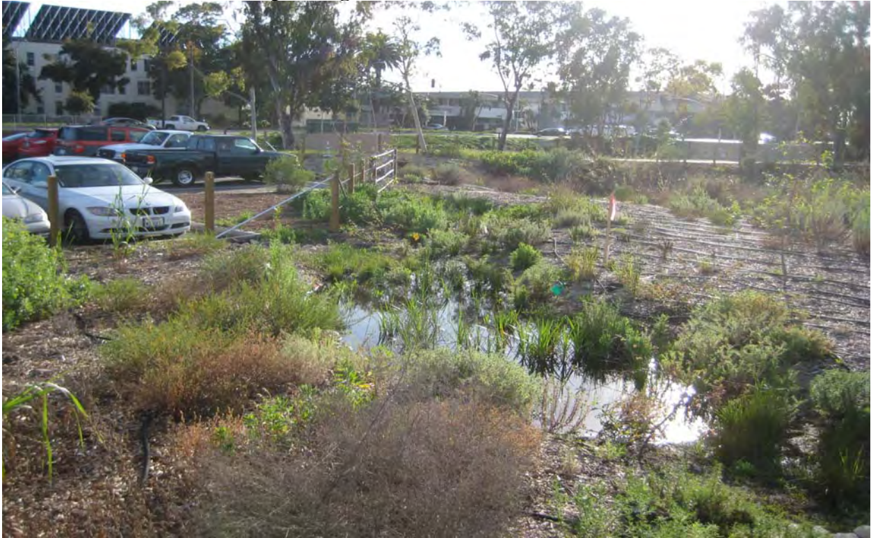
Photo 22. Bioswale #3 flooded during a storm event
