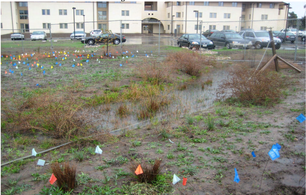
Photo 22. Bioswale #3 flooded during a storm event
