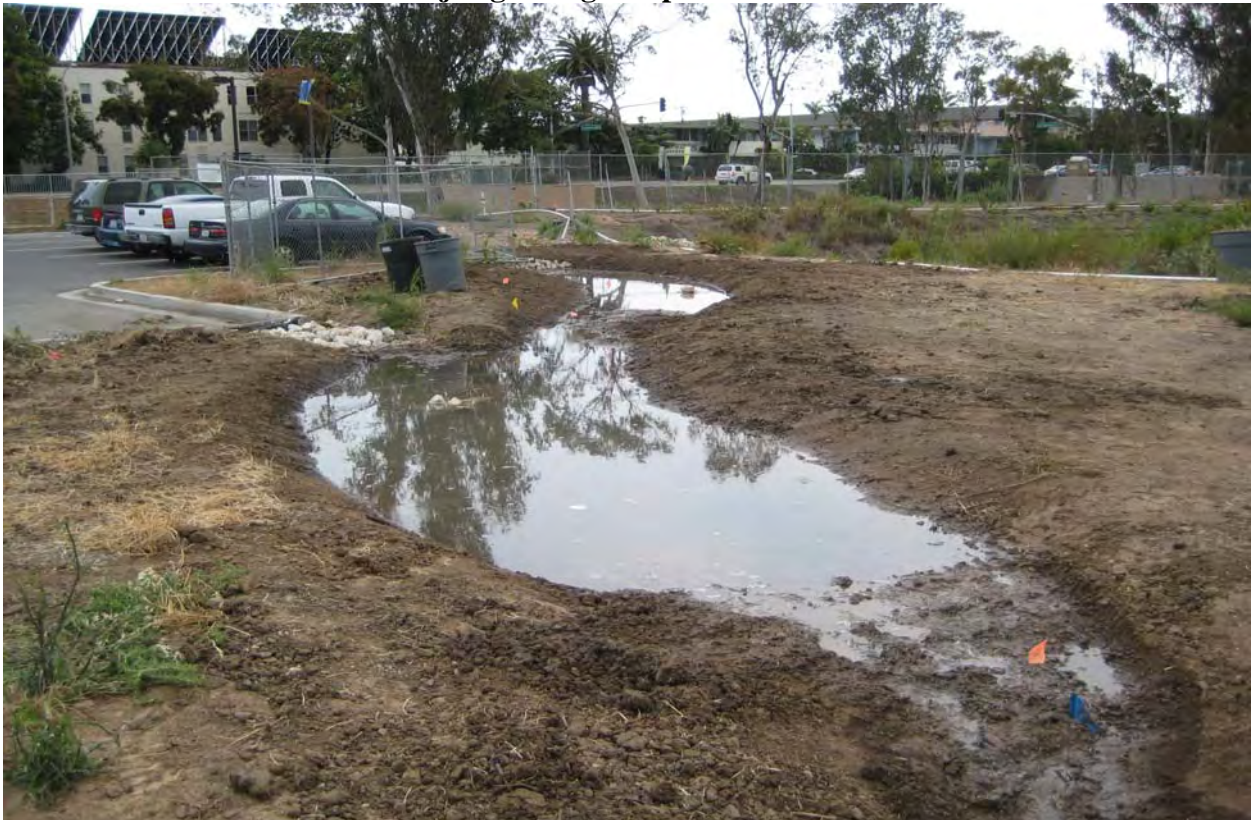
Photo 20. Bioswale # 5 after major grading completed
