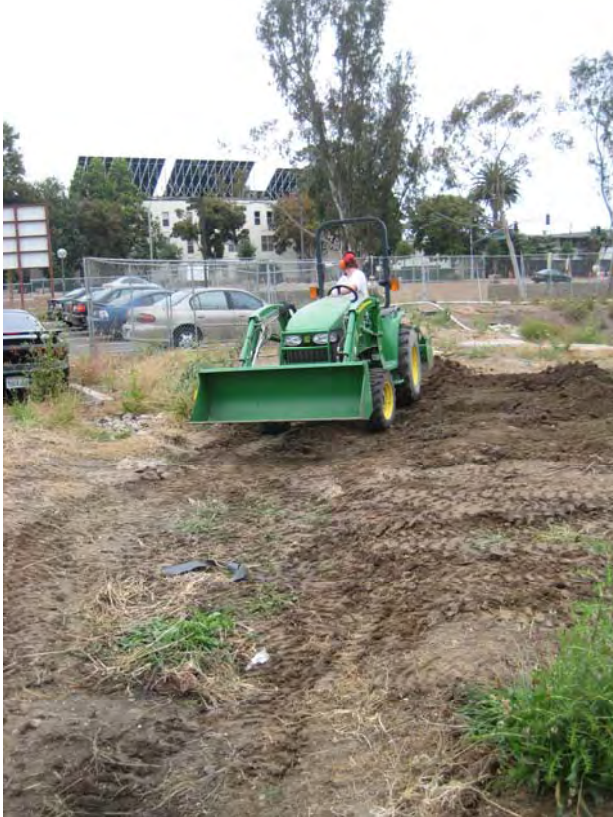
Photo 20. Bioswale # 5 after major grading completed
